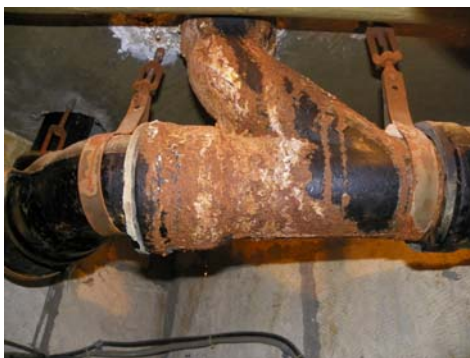
Above: A photo of one the drain pipes that was removed and replaced.
